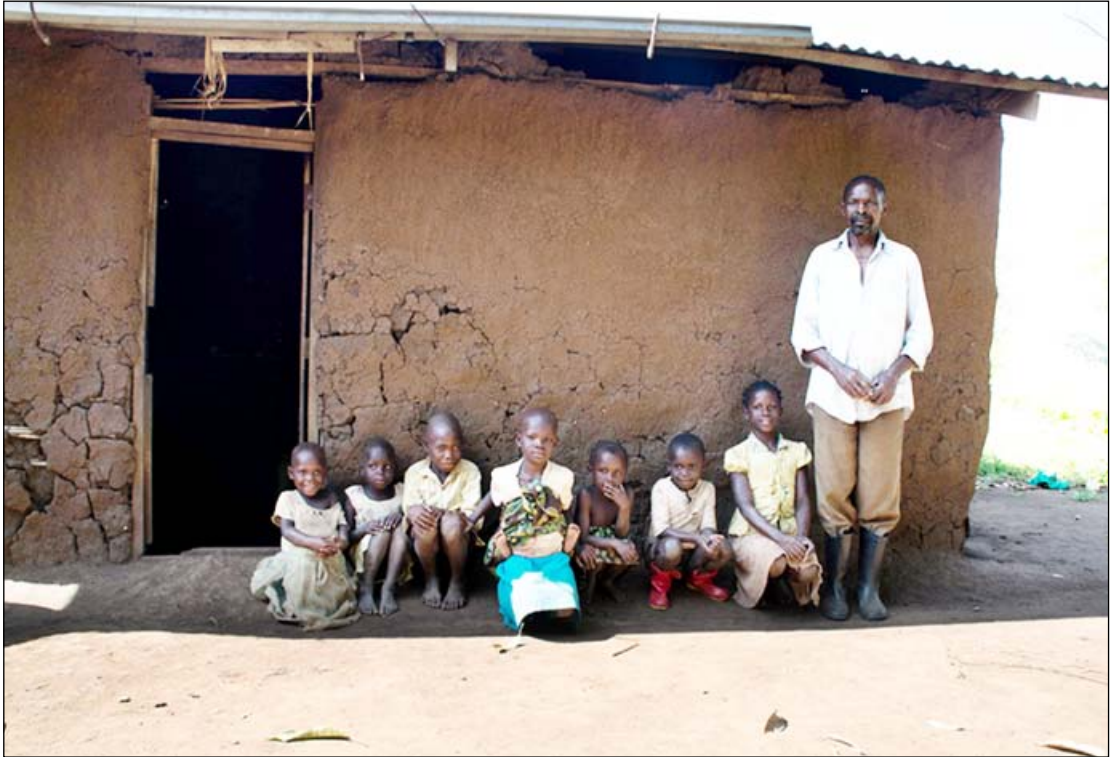
A resident of Howa/Kyenjojo poses in front of his home with seven of his children. This family, living alongside the Hoima Kaiso-Tonya Road, was put in danger during the rock blasting process undertaken to develop the road. Their home and gardens remain damaged today.
