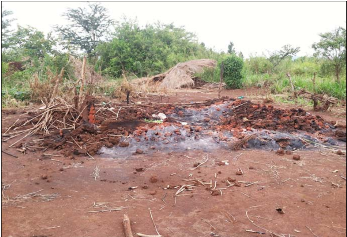
A demolished home inside the boundaries of the disputed territory. Many homes were similarly burnt to the ground and destroyed during the evictions.
